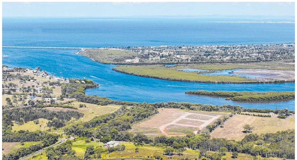
STRONG APPEAL: Unison Projects is unlocking The Shores riverfront section of Griffin Pocket.
